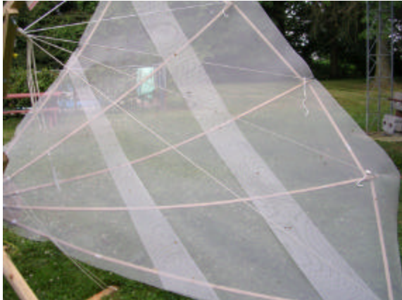
Figure 19. Screening is tie to the struts.
