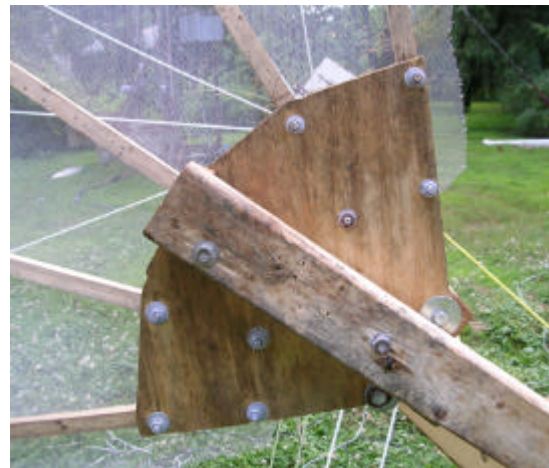
Figure 15. The struts are attached to a square plywood center with two bolts.
