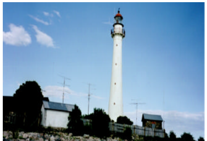
ES8X: 432 EME array is on tower to left of the lighthouse
