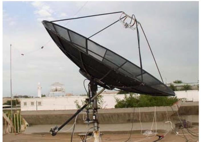
A71AW's 3 m dish used to work HB9Q with 100 W
