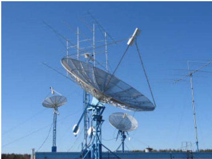
RW1AW's new 6m dish for 23 cm in the foreground with smaller dishes for 13 and 3 cm in the background
