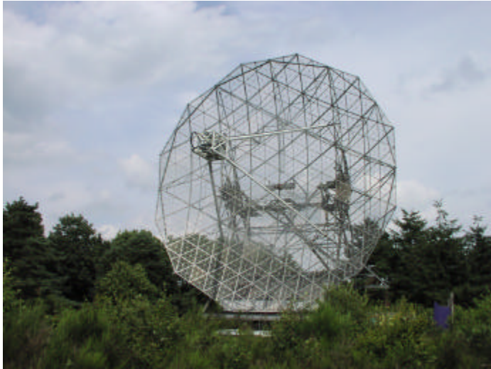
25 m Dwingeloo Radiotelescope coming on 70 and 23 cm EME by CAMRAS group - see PA0PLY's report
