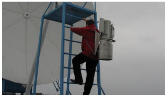
Rocket man, Alex (RW1AW) installing feed on his dish
