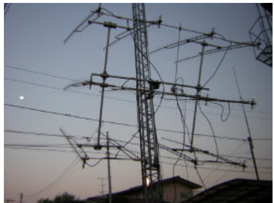
JA0TJU's side tower mounted 12 yagis 70 cm EME array
