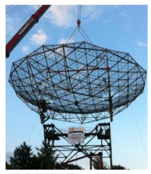
Lift off of PI9CAM 25 m dish for maintenance
