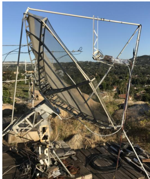
WA6PY's new 6 cm SSPA mounted at dish
