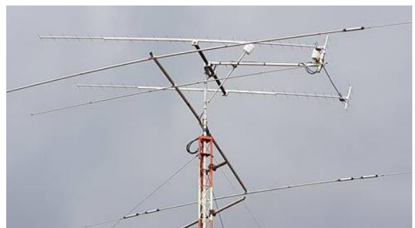
S51LF's 70 cm antenna consists of 2 x 30 el DJ9BV
