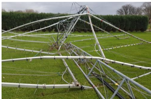
ON4IQ & ON4GG's smashed 432 EME array
