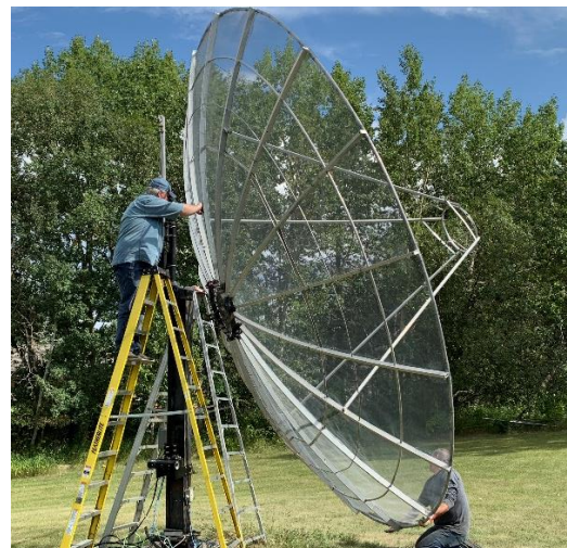
VE6TA's new AZ slewing gear drive being installed – see Grant's report
