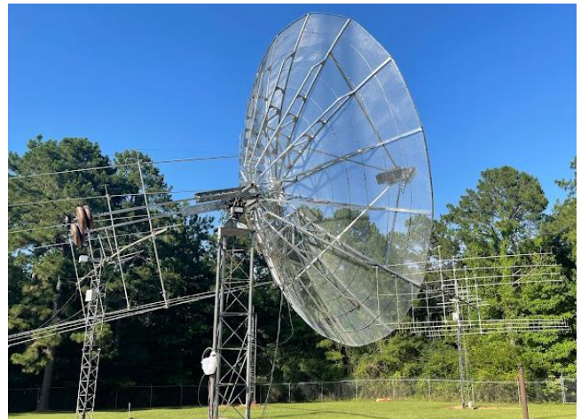
K5QE 6 thru 1296 (including 222) EME antenna farm
