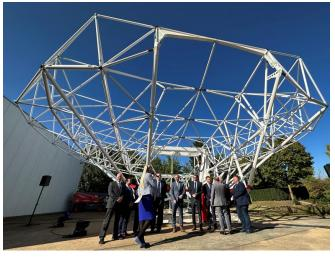
The prototype antenna's 18-meter dish, just under the height of a six-story building, is composed of 76 individual aluminium panels assembled in a striking 8-sided shape. "This design allows the surface of the dish to withstand whatever the environment throws at it—extreme temperature, wind, gravity - the reflector
